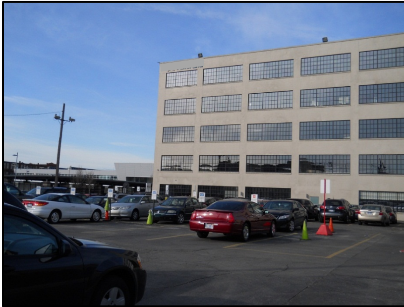
Figure 7 Exterior View of TechHouse
